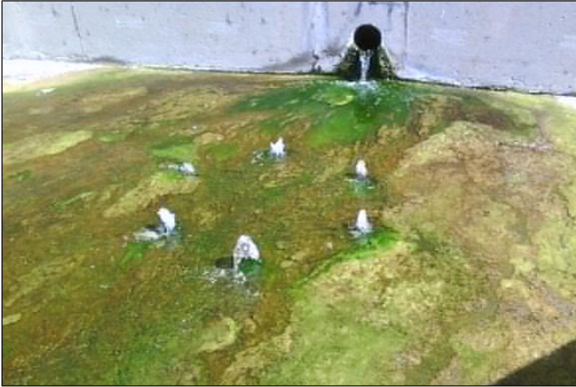
Figure 2. Manhole Exuding Groundwater into San Jose Creek
